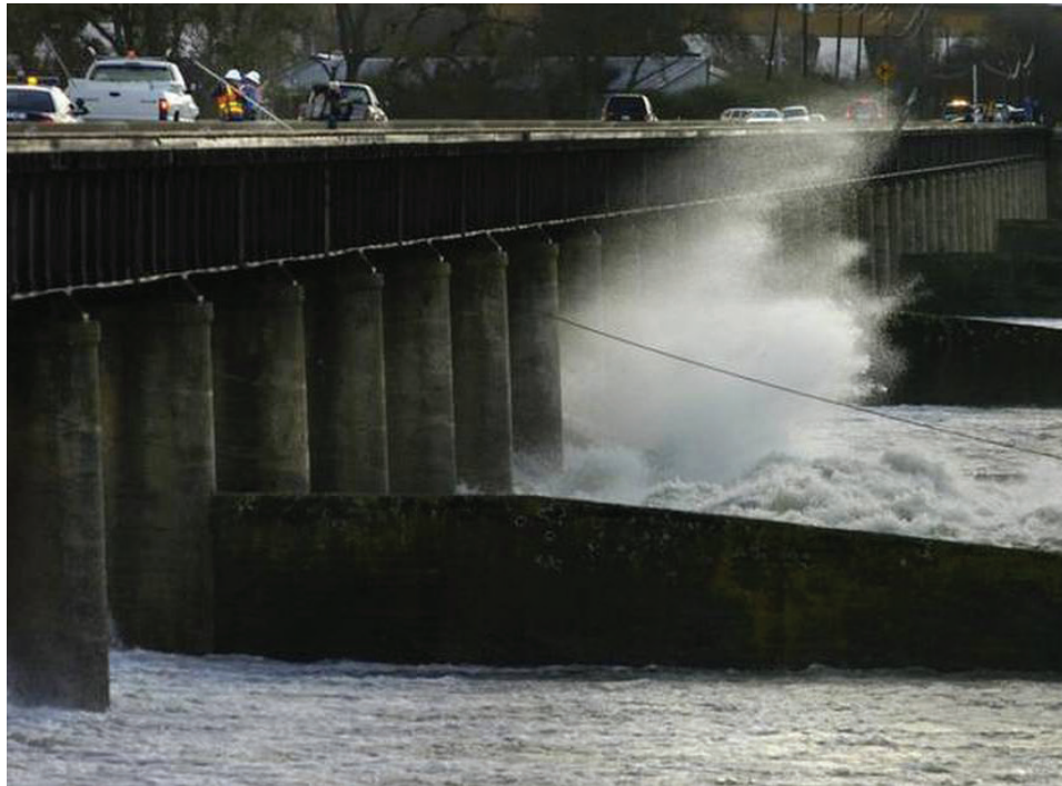
Online Water rushes through the gates of the Sacramento Weir allowing water to flow into the Yolo Bypass. Diverting the water into the Yolo Bypass reduces the water levels on the Sacramento River. Lezlie Sterling Sacramento Bee Staff Photo
